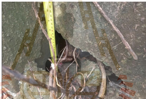
Figure 4.15 Opening due to soil flew out of the bridge approach slab
