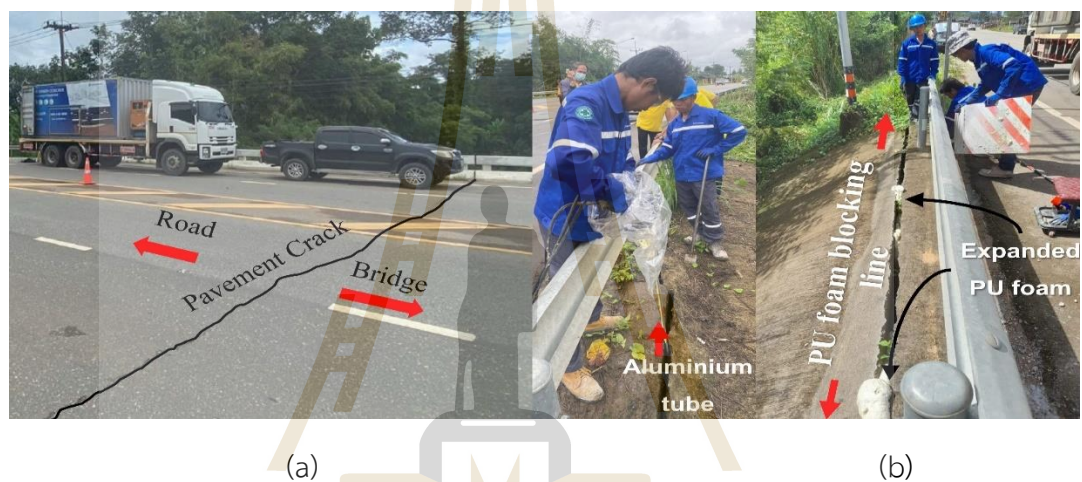
Figure 4.16 (a) Pavement crack line (b) Injection to seal the opening.
