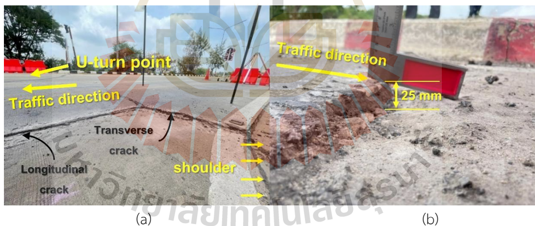
Figure 4.10 Physical characteristics of the road (a) pavement damage (b) settlement surface
