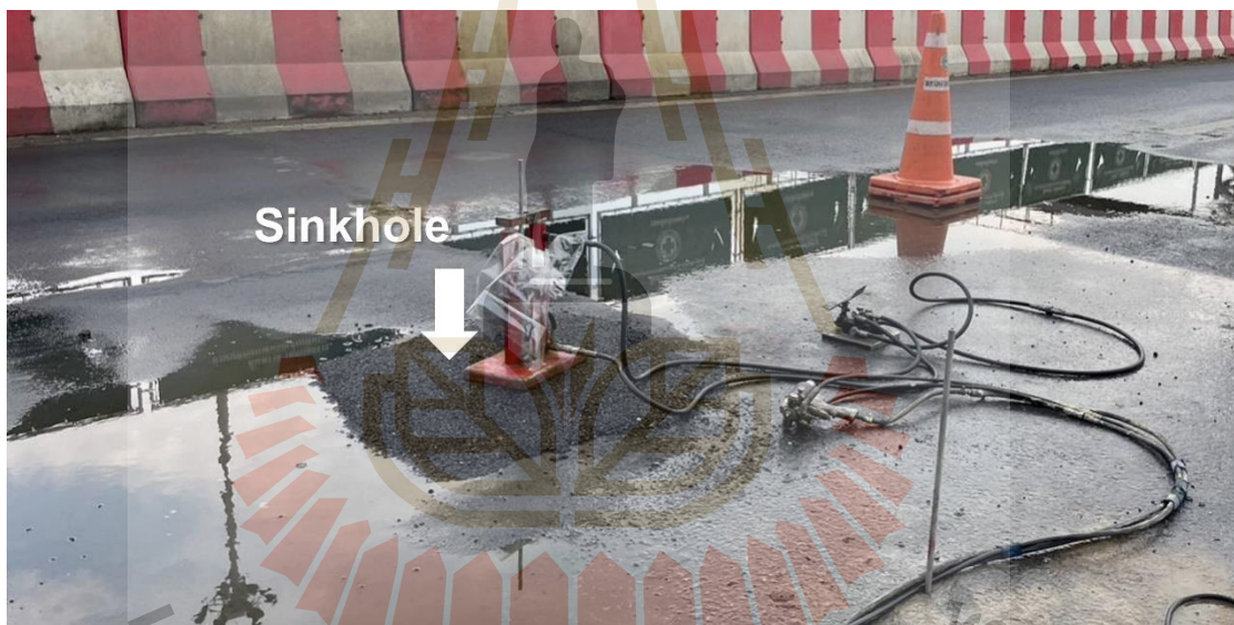
Figure 4.6 Settlement location of the asphalt-covered pavement.
