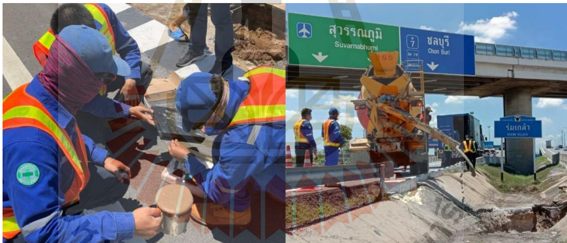
Figure 4.20 Preparing Lightweight concrete for pouring to fill a cavity
