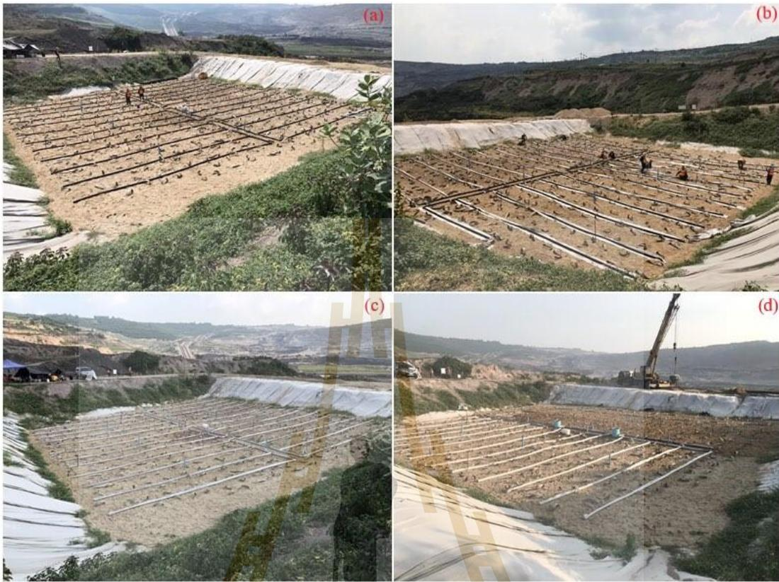
**Figure 5.6** Installation of Neodrain pipes on 30 September 2019: (a) Step 1: Installing Neodrain pipes; (b) Step 2: Preparing geotextile to wrap the pipes; (c) Step 3: Wrapping the pipes by using geotextile; (d) Step 4: Connecting the pipes with the tanks
