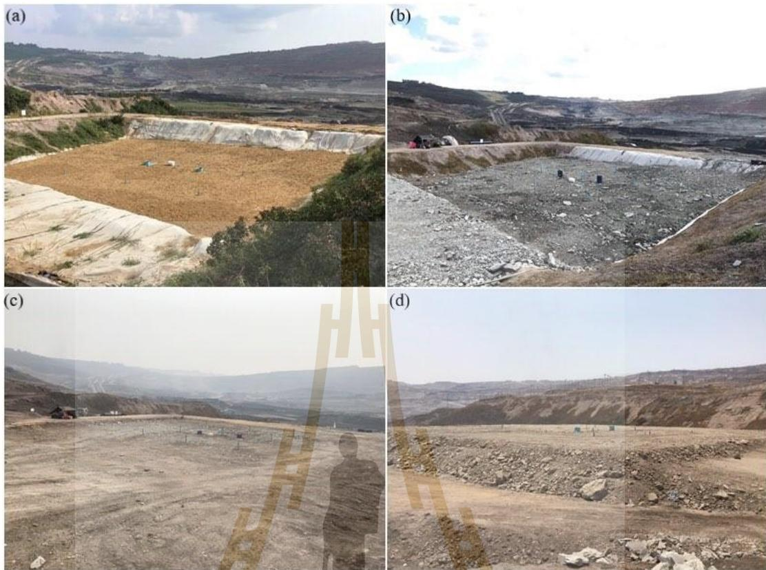
**Figure 5.8** Photos of trial pond after finishing construction of each loading stage: (a) Sand blanket; (b) Loading stage 1: 1.0 m clay stone; (c) Loading stage 2: 1.5m clay stone; (d) Loading stage 3: 2.5 m claystone.
