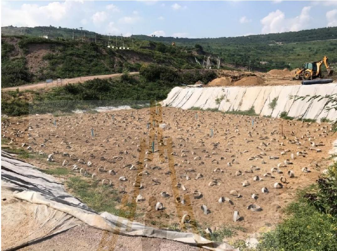
**Figure 5.5:** Completion of PVDs installation on 3 August 2019
