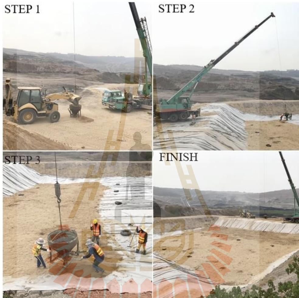
**Figure 5.4** Construction procedure for platform
