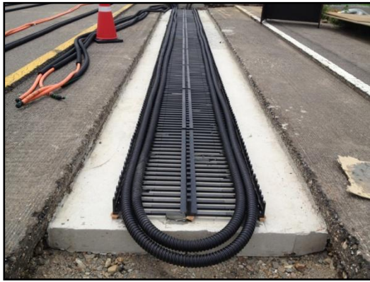
Fig. 1 KAIST OLEV Project (Underground coil segmentation embedded in road)
