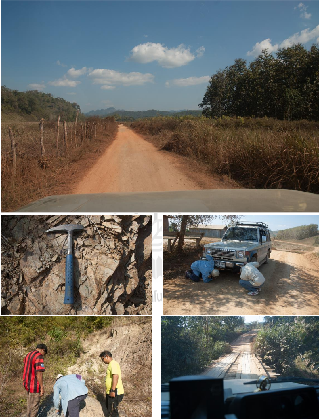
Figure F-4.1 Road condition along the way from Paklay town to Paklay dam site.
