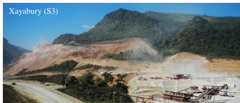
Figure 5.9 Available limestone quarries and the crushing mill located next to the southwest of dam site.
