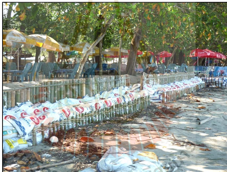
Figure B-7 Small seawall in Hat Pak Meng (taken on 21/7/2555).
