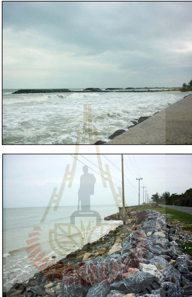
Figure A-26 Breakwaters and seawall along road number 4013 (taken on 19/07/2012).
