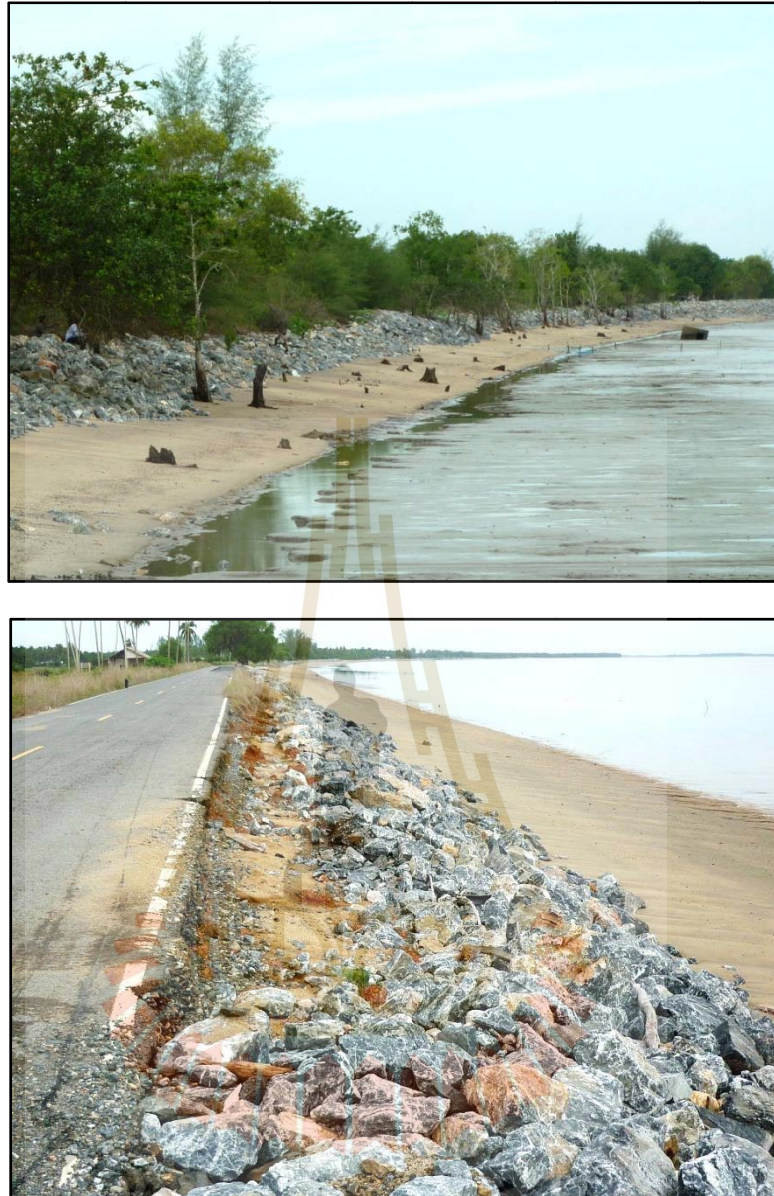
Figure B-14 Seawall in Ban Pak La Ngu area (taken on 20/07/2012).
