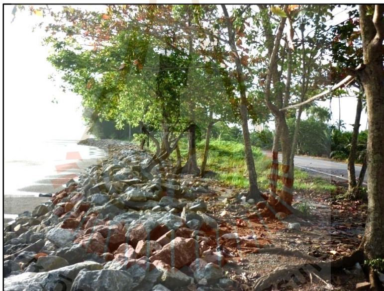
Figure B-11 Seawall in Ban Thung Sabo (taken on 20/07/2012).
