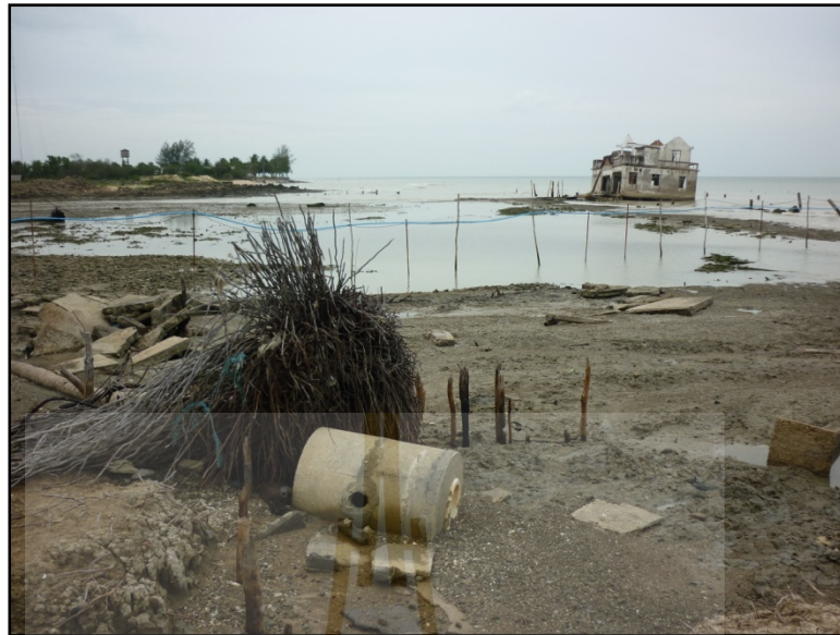
Figure 2.6 Coastal erosion in Ban Tha Praya, Pak Panang District, Nakhon Si Thammarat Province (WGS84 UTM 639975E 914064N).
