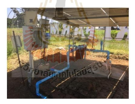
Figure B-2 Water pump and electrical equipment.
