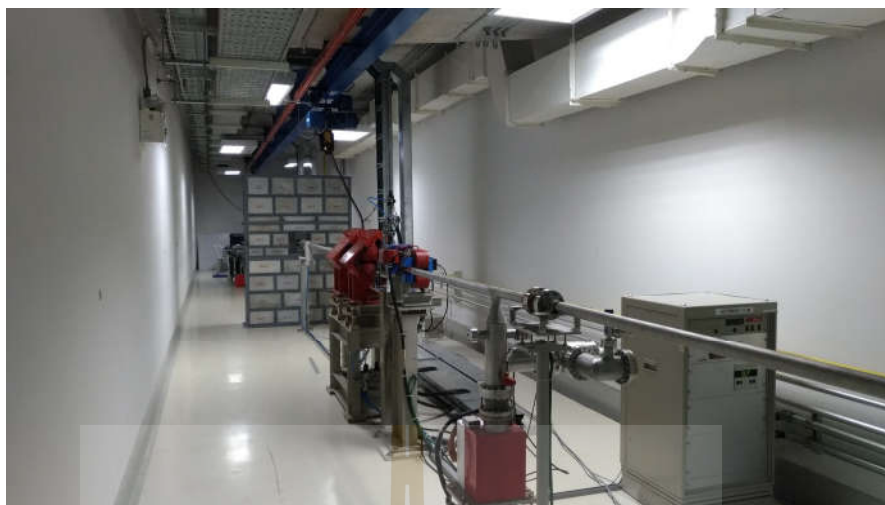
Figure A.4 High-energy Beam Transport at Synchrotron Light Research Institute.
