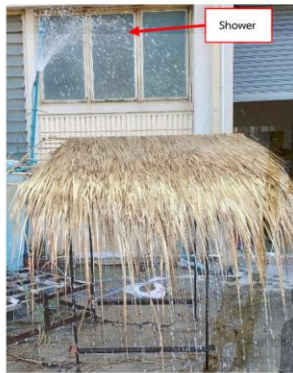
Figure 10 Leakage test by shower.
