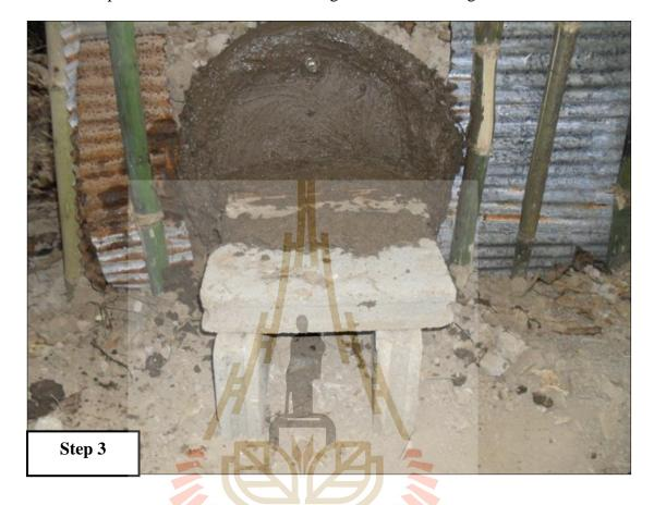
Figure 2.3 Preparing burning gate (An Introduction to Wood Vinegar, 2013).
