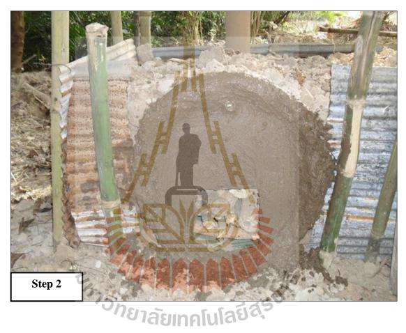
Figure 2.2 Sealing the cover of the kiln (An Introduction to Wood Vinegar, 2013).
