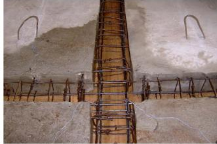
Figure 3 Loop joint connection
