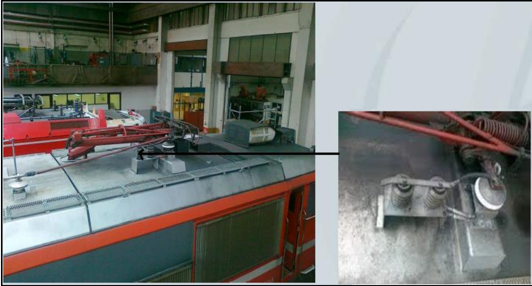
Figure 2.27 Installation of MO surge arrester on locomotives (Pešič, and Grmovšek, 2007).
