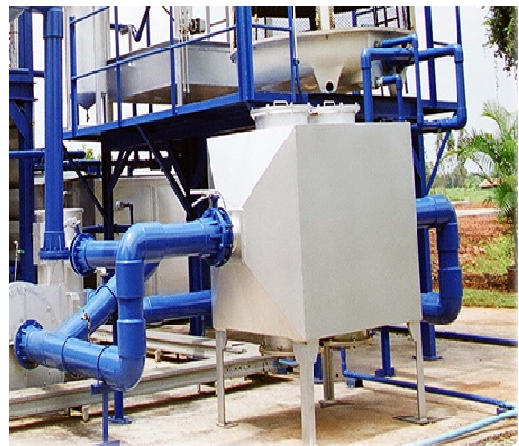
ฉ. Biomass Filter Unit
