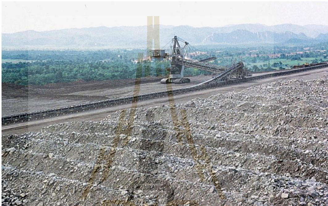
Figure 1.2 Transporting the waste dump materials to the disposal area using a conveyor system.
