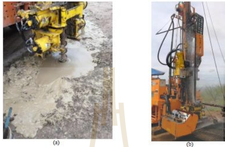
Figure 7 Photos of representative borehole installation: (a) At the first bench; (b) At the B-3 borehole
