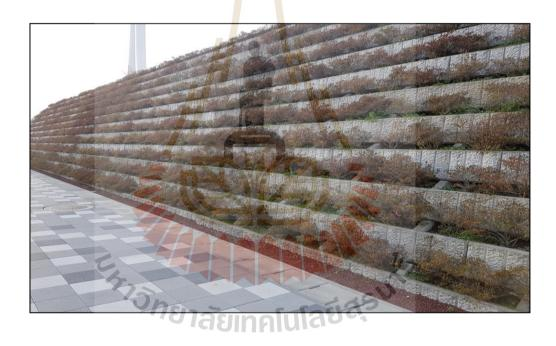
Figure 2.5 Typical prefabricated modular walls
