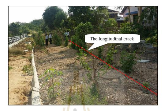
Figure 5.4 The longitudinal crack along the wall facing of the riverbank protection structure.
