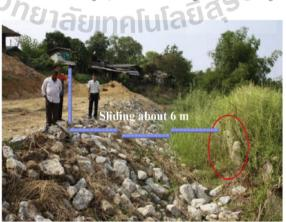
Fig. 1. Large movement of wall facing of the first riverbank protection structure.
