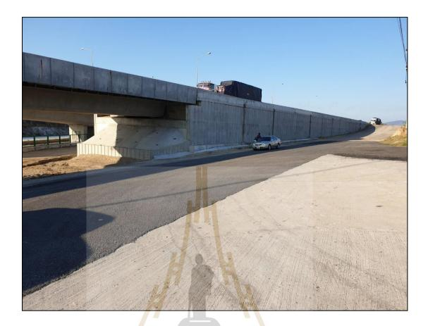
Figure 2.4 Typical semi-gravity retaining walls
