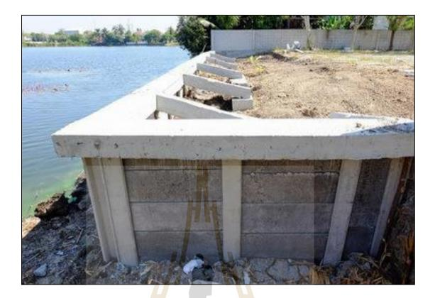
Figure 2.3 Typical semi-gravity retaining wall
