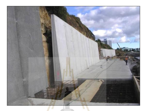
Figure 2.1 Typical semi-gravity retaining walls
