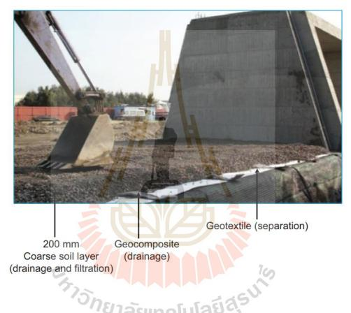
Figure 2.14 Wall construction with 200 mm thick layer of coarse soil cushion above drainage layers to placing of locally available backfill soil (Thuo et al. 2015).
