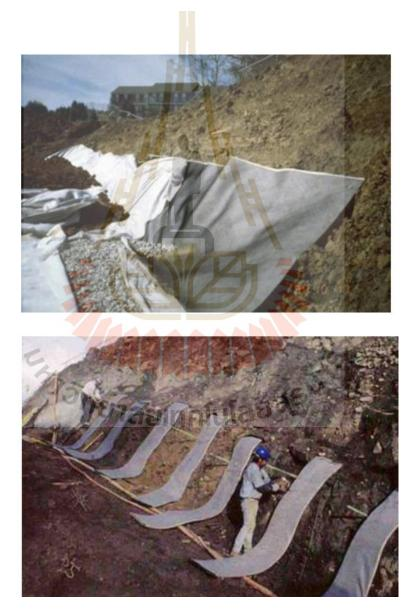
Figure 2.6 Back drainage set up behind MSE walls (Koerner et al. 2011).
