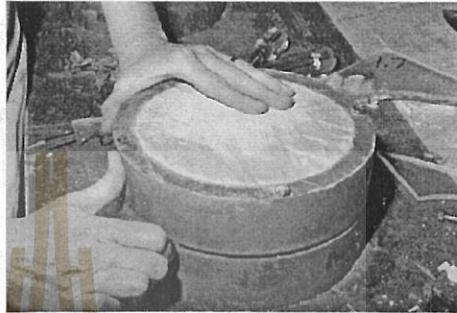
FIG. 7 Removing Spacer Plates After Encapsulating Material Has Cured
