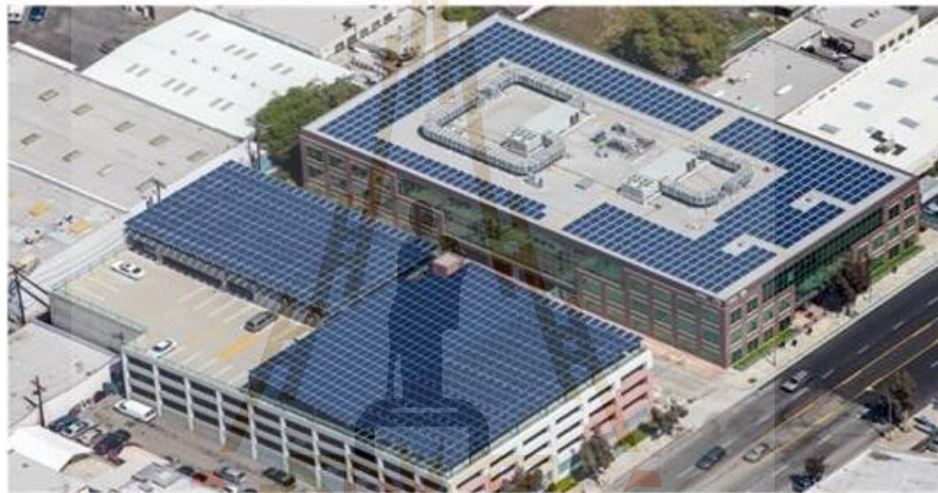
Commercial Roof-Top PV System - Glendale 342 kW Solar System
