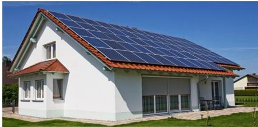
Residential Roof-Top PV System - Berkley Residential PV System
