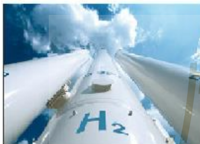
Hydrogen Energy Storage System
