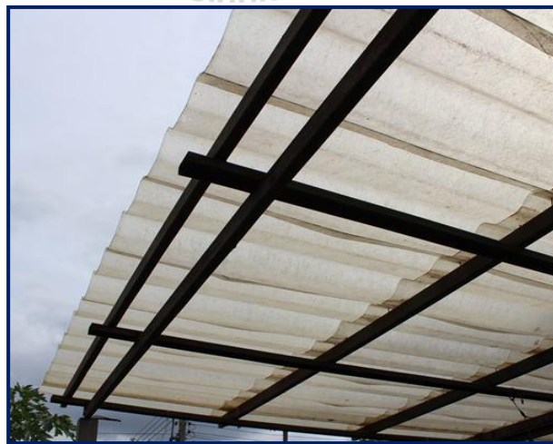
Figure 3.5 Transparent roof above the constructed wetlands.
