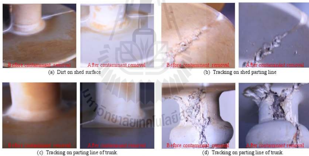
Fig. 6 Surface damaged of Type-B specimens
