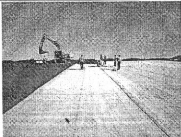
comprised of sodium bentonite, bound by a woven and non-woven geotextile or adhered to a geomembrane.
