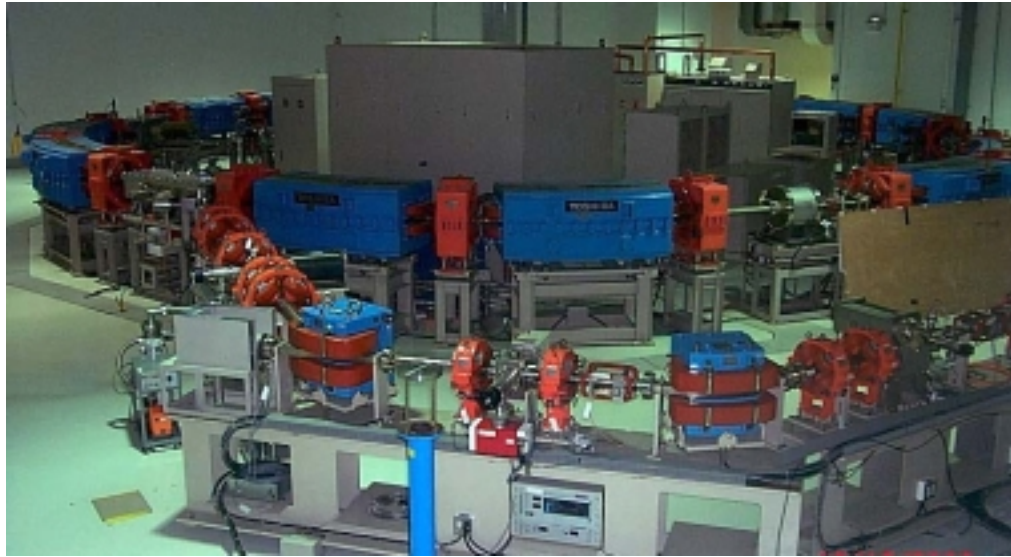
Fig.1.3 A Low-Energy Beam Transport Line (LBT) and Booster Synchrotron (SYN)
