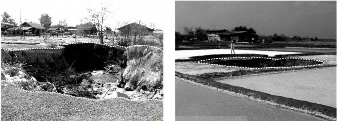
**Figure 2.2** Brine pumping operation cause the sinkhole in Sakon Nakhon basin
