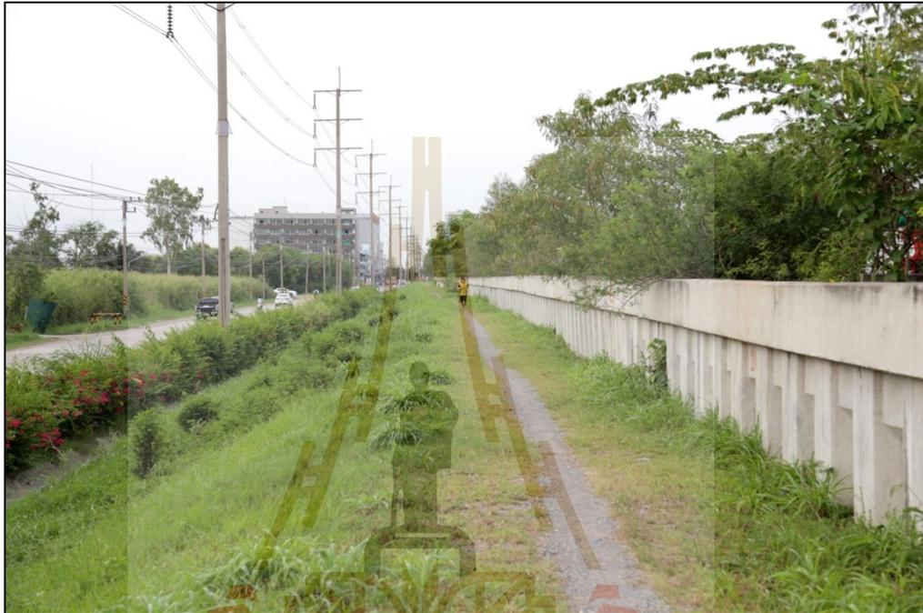
**Figure 2.2** Typical Non-gravity cantilevered retaining walls
