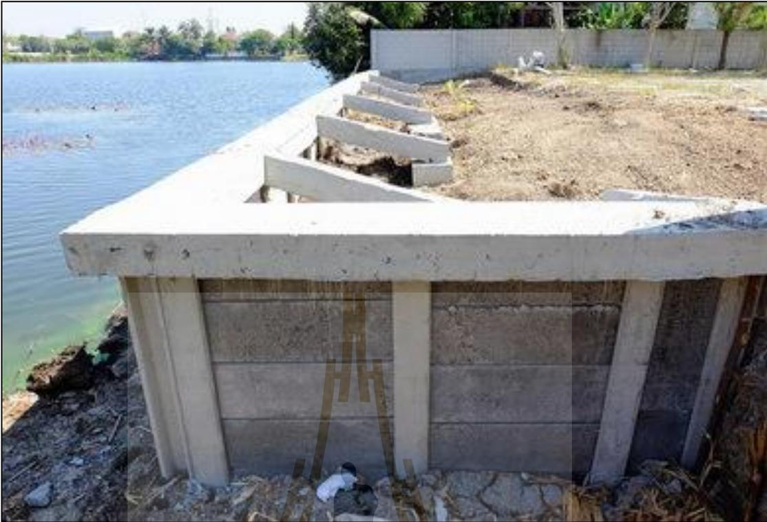
**Figure 2.3** Typical semi-gravity retaining wall
