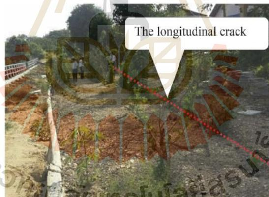
Fig. 4. The longitudinal crack along the wall facing of the riverbank protection structure.
