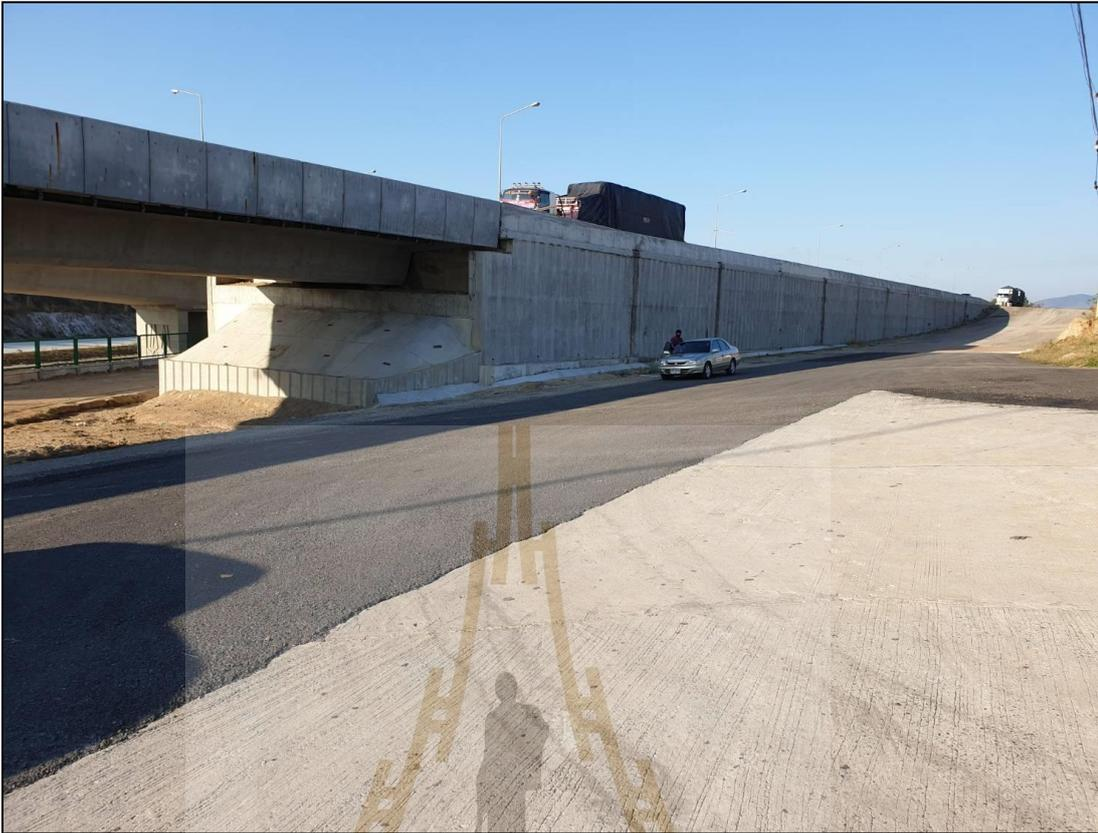
**Figure 2.4** Typical semi-gravity retaining walls
