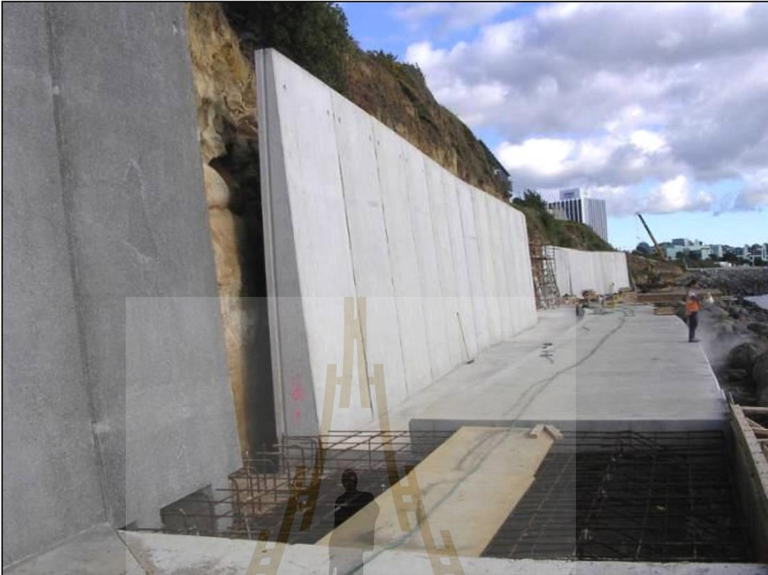
**Figure 2.1** Typical semi-gravity retaining walls
