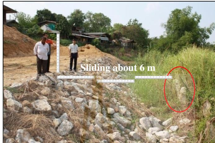
**Figure 5.1** Large movement of wall facing of the first riverbank protection structure.
