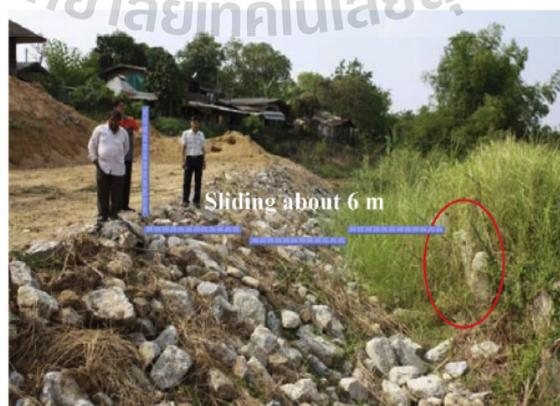
Fig. 1. Large movement of wall facing of the first riverbank protection structure.
