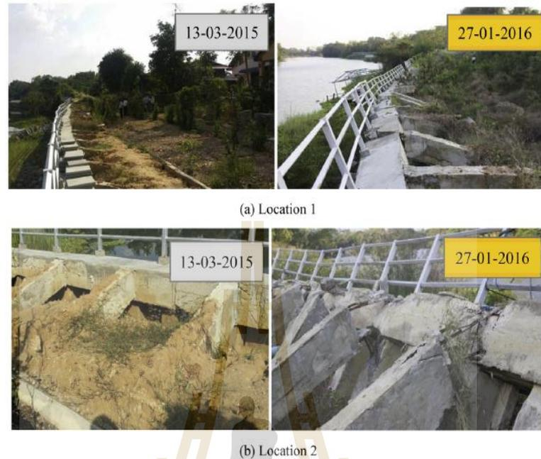
Fig. 3. The retaining walls before and after its failure at: (a) Location 1 and (b) Location 2.
