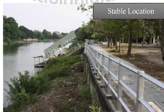
Fig. 7. The visual observation of the stable retaining wall structure.
