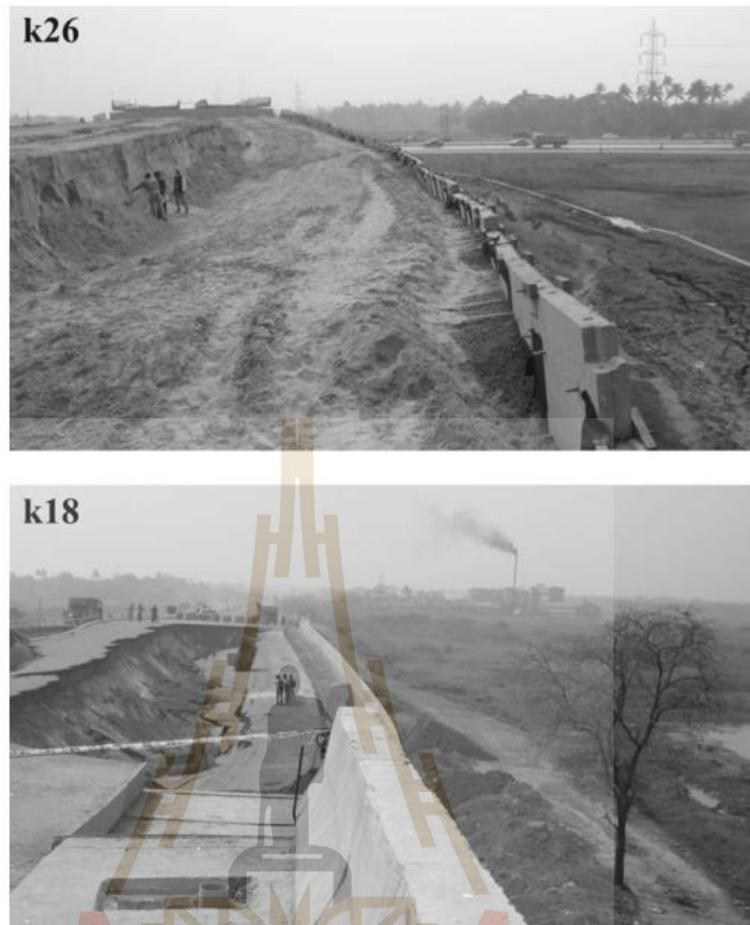
**Figure 2.49** MSE Failures at research area in Roy and Singh 2008.
