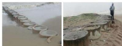
**Figure 6.** Column - shaped reinforced dyke for embankment protection (Xuan Hoi - Xuan Pho) and anti - accumulation at Hoi estuary.
