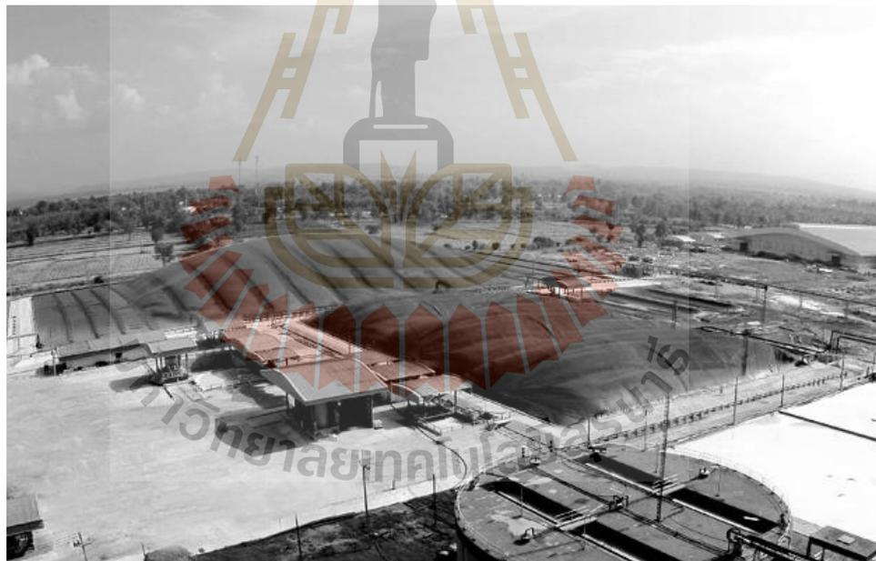
**Figure 3.1** The modified covered lagoon (MCL) from a cassava starch factory.
