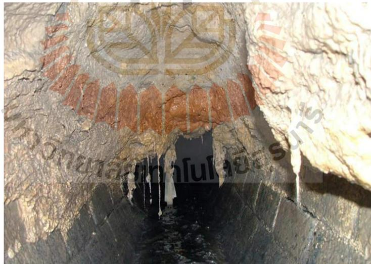
**Figure 2.1** FOG deposit turning into a “fatberg” in the sewer system (Thames Water, 2017).
