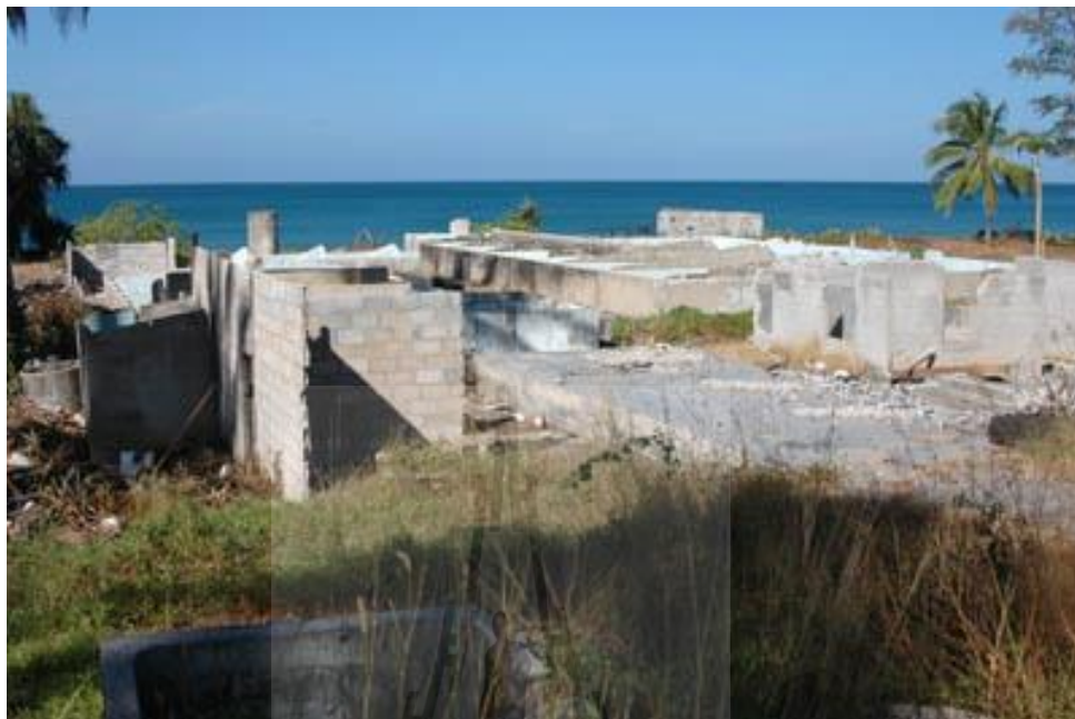
Figure 2.17 Shrimp hatcheries were damaged (FAO and MOAC, 2005).
