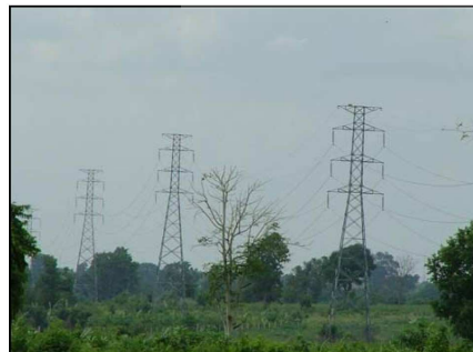
Fig. 2 Electric power transmission line in Nakhon Ratchasima
