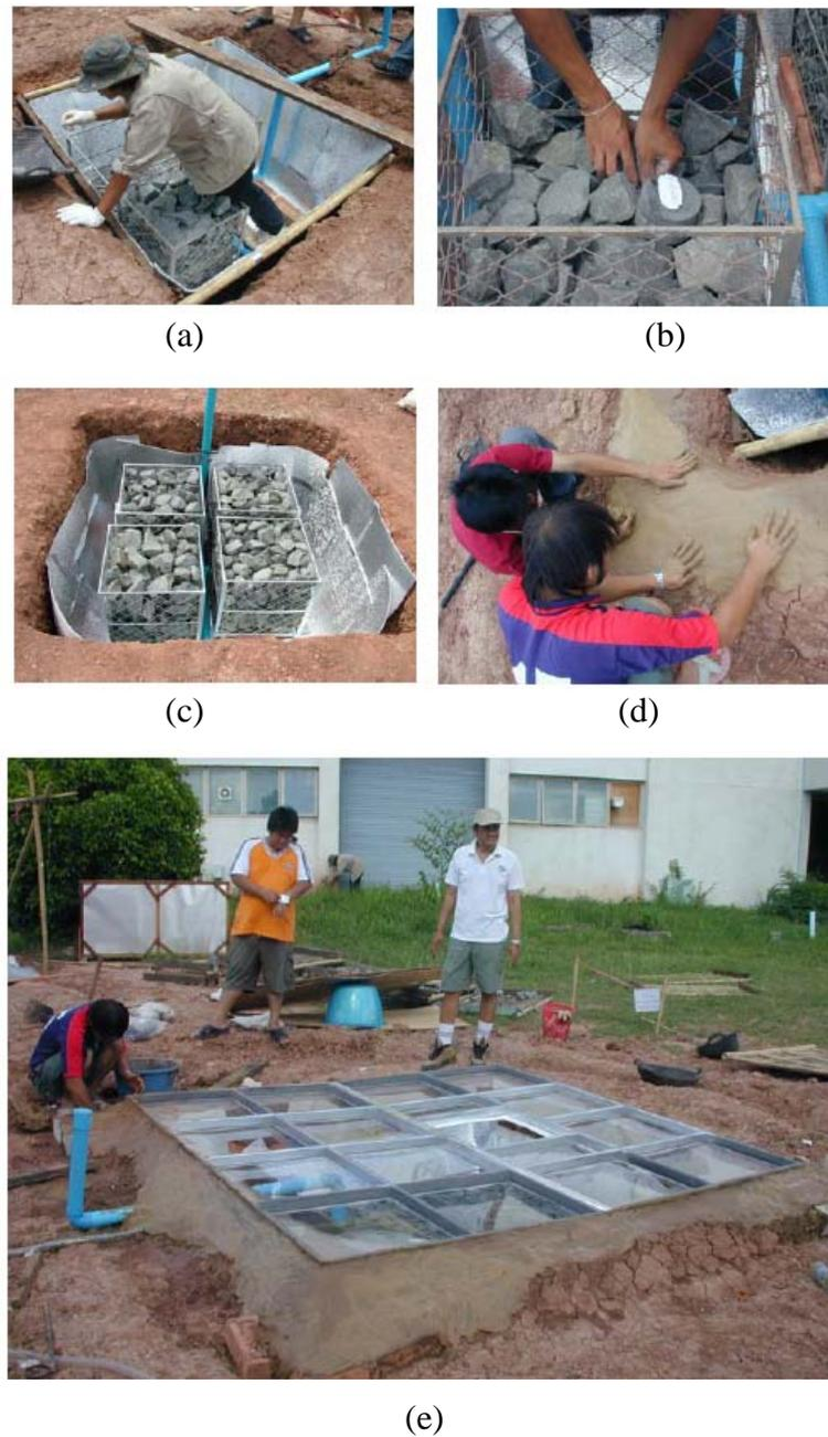
**Figure 5.3** Storage pit construction: (a) placing of rock baskets, (b) packing rock fragments in the baskets and installing thermocouples, (c) placing insulator sheets around pit walls and floor, (d) shaping the pit rim with clay, and (e) installing acrylic sheets reinforced by steel frames.
