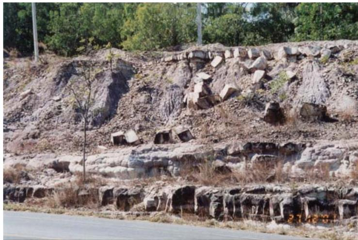
**Figure A.14** The block sizes of sandstone are  $0.7 \times 0.8 \times 0.5 \text{ m}^3$  at the toe of slope (slope no.3).
