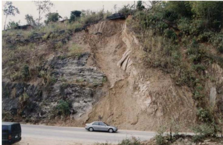
**Figure A.94** The failure of slaty-shale slope is located at km 36 to 37 of highway no.12, Chum Pare district, Khon Kaen province (slope no.33).
