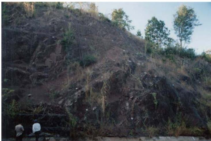
**Figure A.84** The modes of failure are combination of plane and wedge sliding on the siltstone slope (slope no.29).
