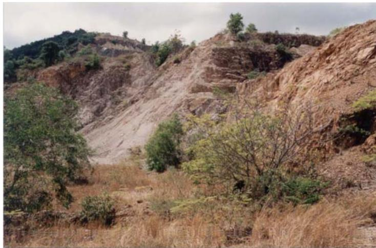
**Figure A.24** Circular failure of blocky rock slope of slaty-shale quarry, Chon Buri province (slope no.10).
