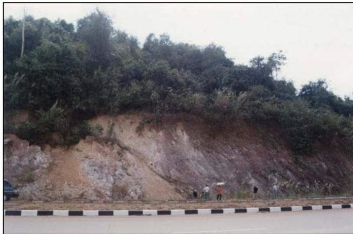
**Figure A.19** The circular failure of heavily jointed rock slope on highway no. 344, Chon Buri province (slope no.7).
