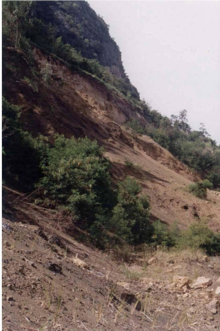
**Figure A.9** The excessive excavation of the soft shale formation at the toe of Khao Chow Lai Yai (slope no.2).
