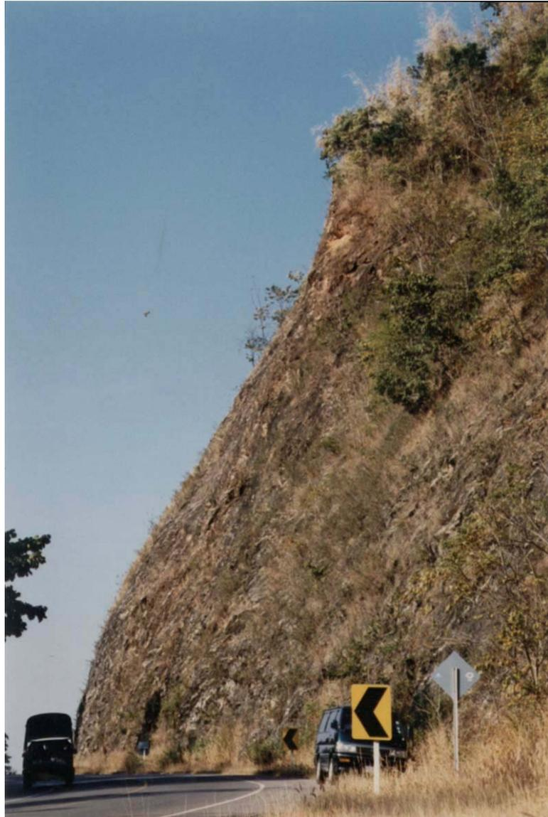
**Figure A.89** The stable slaty-shale slope is located at km 17 to 18 of highway no. 12, Lom Sak district, Petchabun province (slope no.31).
