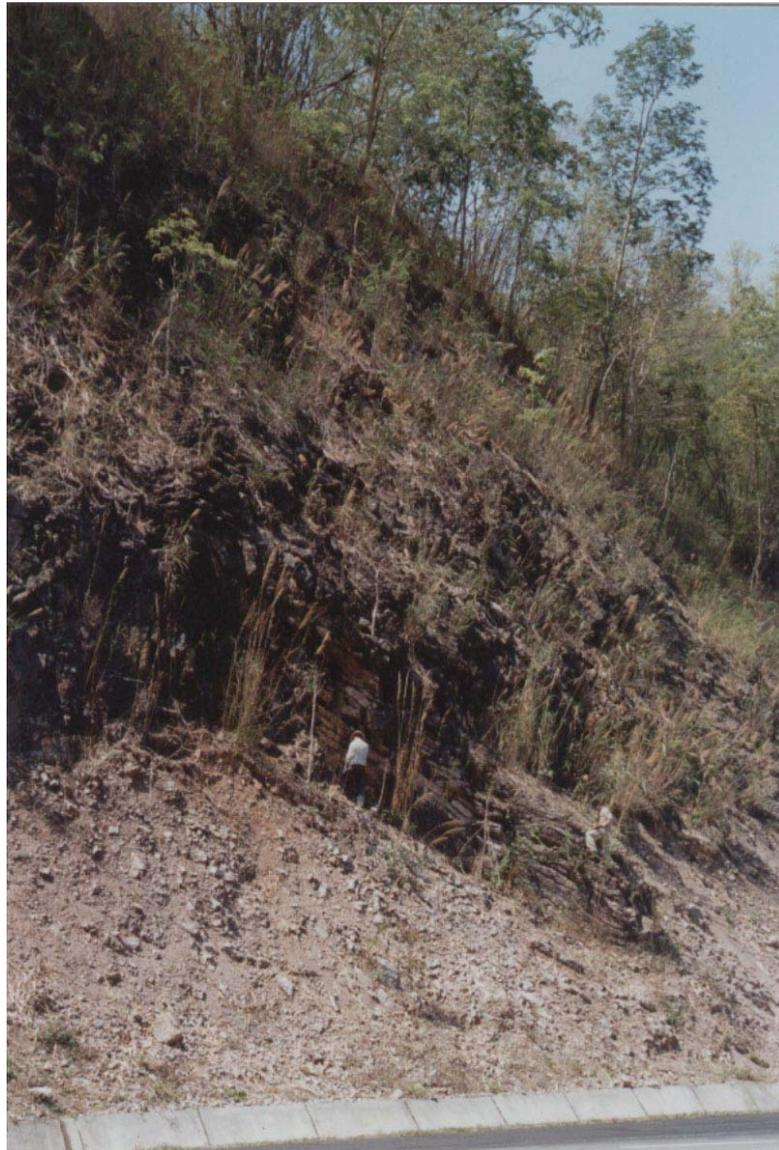
**Figure A.117** The heavily jointed rock at km 49-50 of highway no.105,
