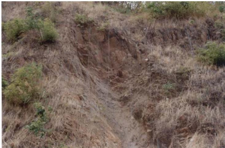
**Figure A.139** The surface failure of shale and wire mesh on slope at km 19-20 of highway no.105, Tak province (slope no.46).
