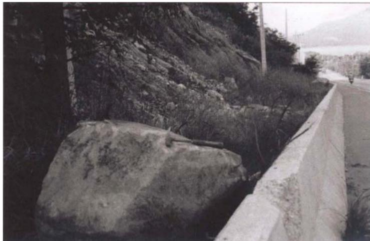
**Figure A.34** Sandstone block size is  $2 \times 1 \times 1 \text{ m}^3$  on the toe of slope (slope no.13).
