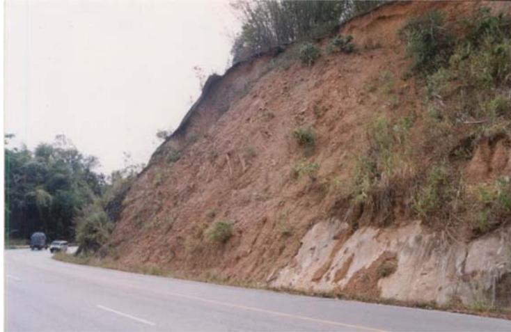
**Figure A.97** The failure of slaty-shale slope is located at km 36+600 of highway no.12, Chum Phae district, Khon Kaen province (slope no.34).
