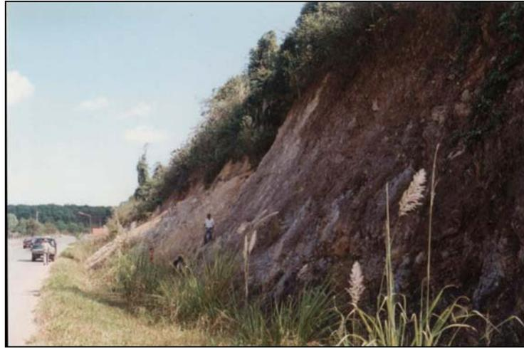
**Figure A.18** Heavily jointed rock slope is located at km 92-93 of highway no.344 (slope no.7).
