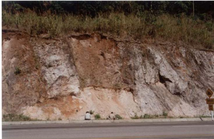
**Figure A.115** The surface circular failure of calcareous shale at km 62-63 of highway no.105 (slope no.38).
