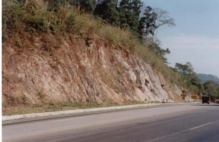
**Figure A.114** The heavily jointed rock at km 62-63 of highway no.105, Mae Sot district, Tak province (slope no.38).
