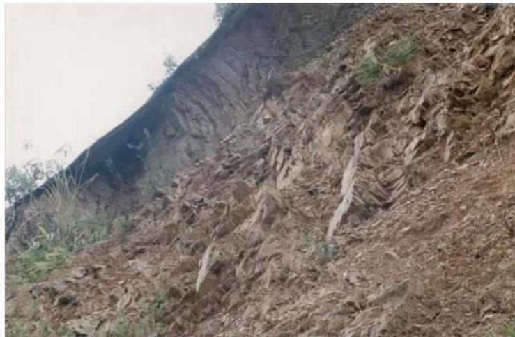
**Figure A.98** Rock slope at km 36+600. Failure surface exposed after massive slope failure. The failure brought down both earthen and installed materials. The remaining shotcrete appears on the left side of the slope face (slope no.34).
