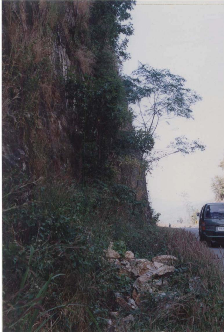
**Figure A.68** The falling rock of limestone at the toe of slope (slope nos. 24 and 25).
