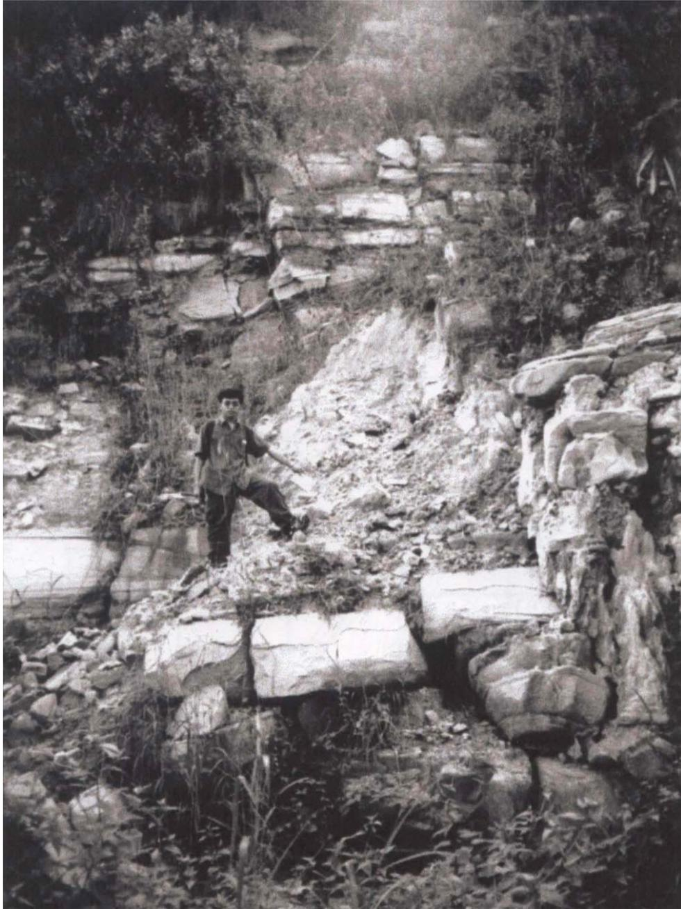
**Figure A.37** The failure is caused by the erosion of the soft shale bed which results in the collapse of the hard sandstone bed (slope no.14).
