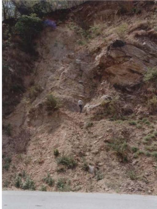
**Figure A.125** The toppling failure of schist slope 21-22 of highway no.105 Tak province (slope no.42).
