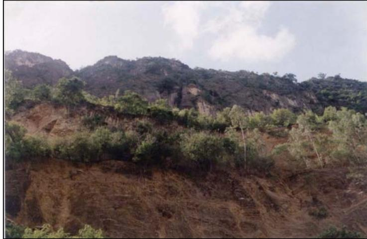
**Figure A.8** The excessive excavation of the soft shale formation at the toe of Khao Chow Lai Yai (slope no.2).
