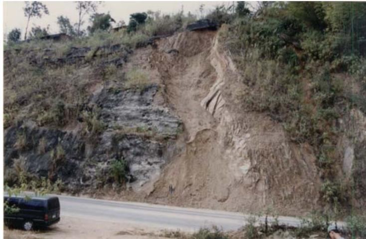
**Figure A.93** The failure of slaty-shale slope is located at km 36-37 of highway no. 12, Chum Pare district, Khon Kaen province (slope no.33).
