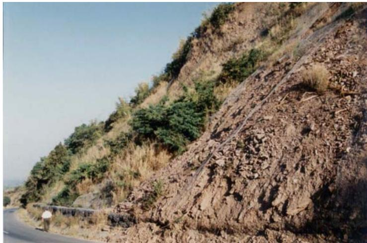
**Figure A.88** The surface failure of heavily jointed rock, Lom Sak district, Petchabun province (slope no.30).
