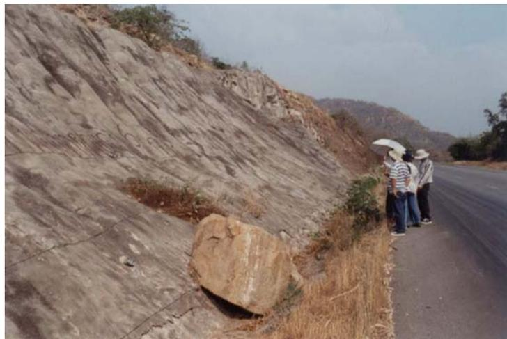
**Figure A.31** The sandstone block size is  $0.8 \times 0.7 \times 0.7 \text{ m}^3$  on the toe of slope (slope no.12).
