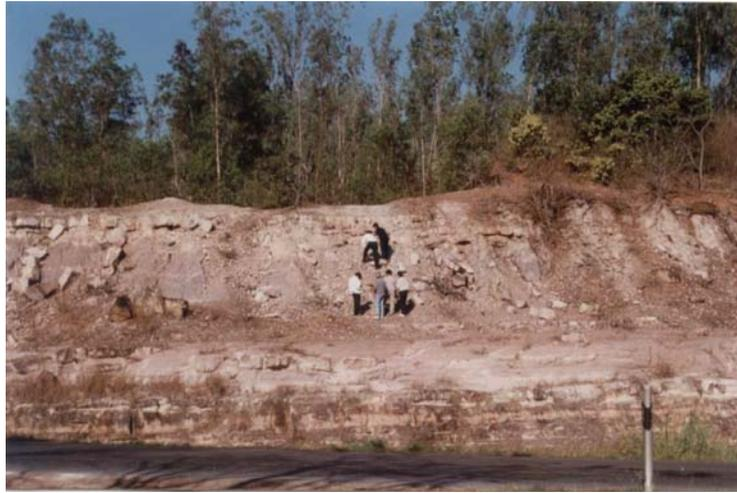
**Figure A.13** The secondary toppling of hard-soft interbedded rock is located at km 70 of highway No. 304 (slope no.3).
