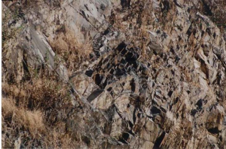
**Figure A.90** Heavily jointed of slaty-shale on slope is located at 17-18 of highway no.12, Lom Sak district, Petchabun province (slope no.31).
