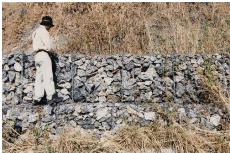
**Figure A.92** Gabion wall at the toe of slope, Lom Sak district, Petchabun province (slope no.32).
