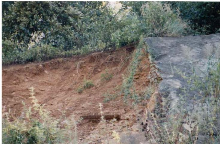
**Figure A.76** The mode of failure is circular on the top of heavily jointed slope (slope no.27).
