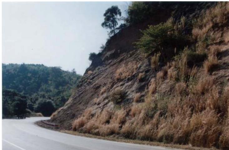
**Figure A.80** The mode of failure is circular on the top of heavily jointed slope (slope no.28).
