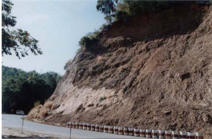
**Figure A.79** The heavily jointed slope is located on 22 to 23-km of highway no.12, Lom Sak district, Petchabun province (slope no.28).
