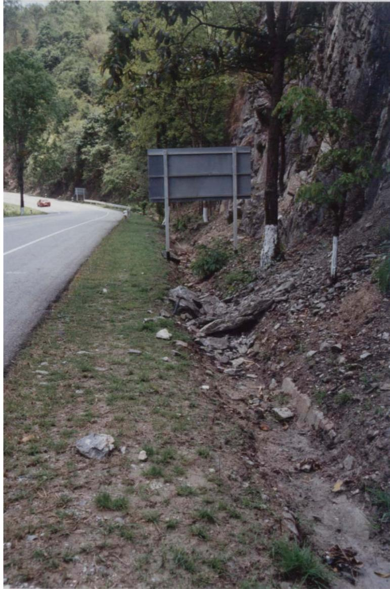
**Figure A.129** Schist slope failure at km 21-22 of highway no.105 (slope no.43).
