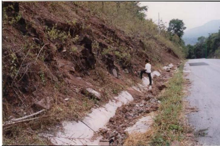
**Figure A102** The size are  $0.15 \times 0.2 \times 0.2$  to  $0.6 \times 0.5 \times 0.3$  m<sup>3</sup> of falling rock at the toe of slope (slope no.35).
