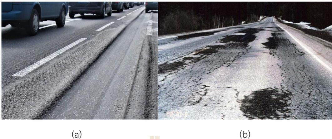
**Figure 2.3** The two main damage characteristics in asphalt concrete pavement (Wang et al., 2021).
