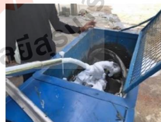
Fig 3. Adding foam agent into mortar
