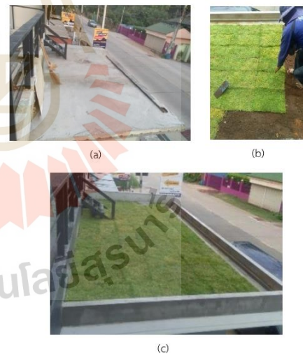
Fig 7. (a) Roof deck from LCC, (b) Planting the vegetation on green roof, and (c) Green roof integrated LCC
