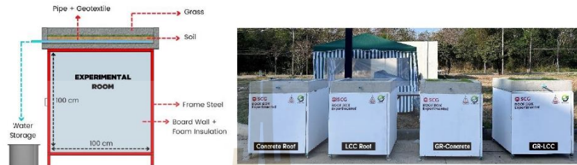
Figure 2. Roof experimental boxes for oncrete roof, LCC roof, GR-Concrete, and GR-LCC
