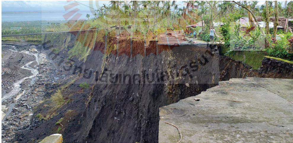
Figure 1.4 Collapsed road at Malilipot, Albay toppled due to erosion dated November 2020 (Photo from The Philippine Examiner).
